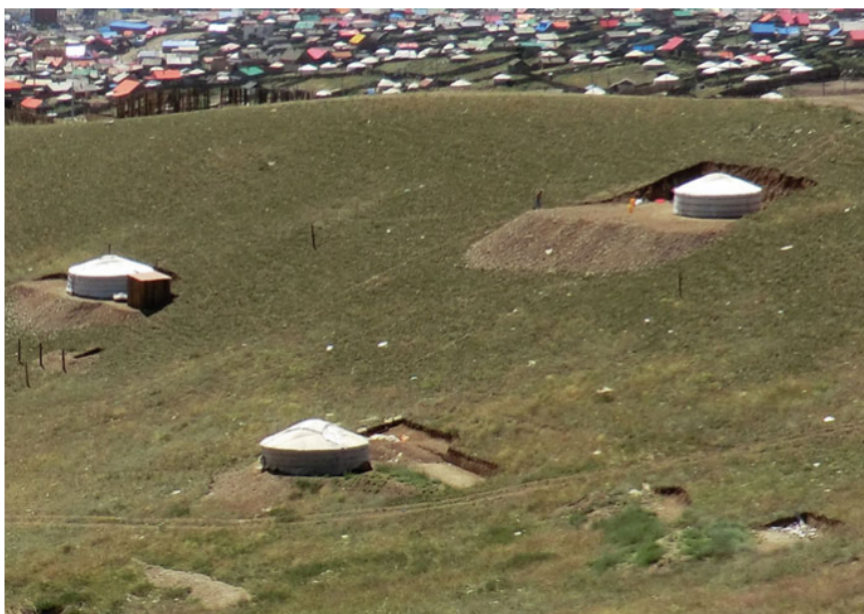
Immagine 5: Construction of gers on steep slopes by digging and developing lands in Ulaanbaatar [Ref. 8 - Saizen, Izuru & Tsutsumida, Narumasa. (2017). The Rapid Development of Settlements in Flood-Prone Areas in Peri-Urban Ulaanbaatar, Mongolia: Monitoring and Spatial Analysis Using VHR Satellite Imageries. 10.1007/978-4-431-56442-3_8.
