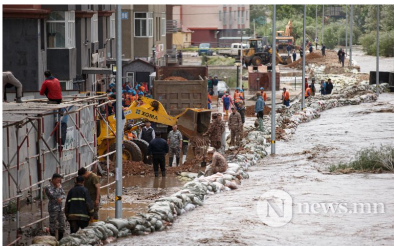
Immagine 8: Building of artificial embankments to contain the flood water in Ulaanbaatar
